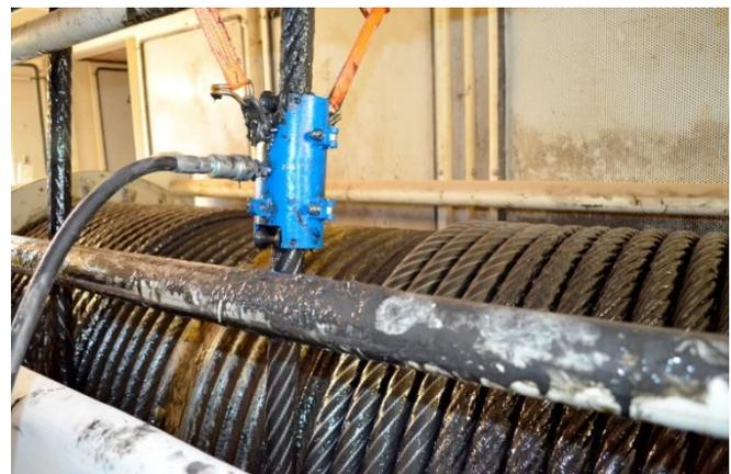
The above are examples of a wire rope lubricators to ensure proper and effective lubrication on wire ropes (picture on the left courtesy of Viper WRL Pty Ltd and on the right courtesy of SKF)
